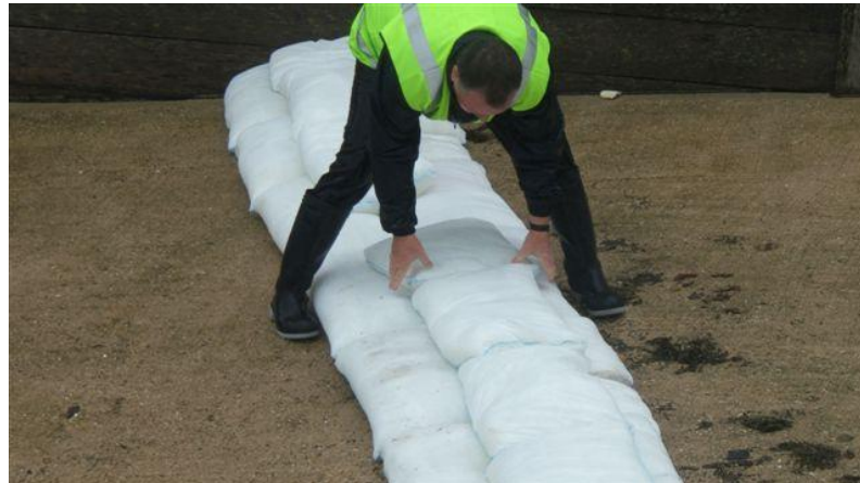
Picture shows inflated bags being placed across the slipway.
